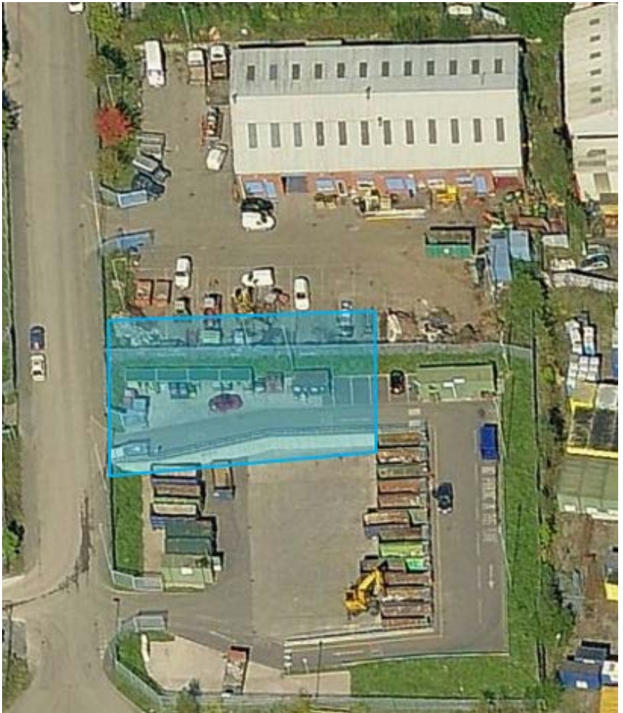
Penallta – Phase 2 Works
