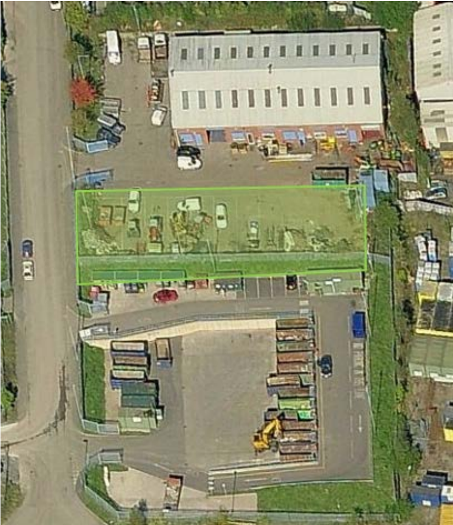
Penallta – Phase 1 Works
